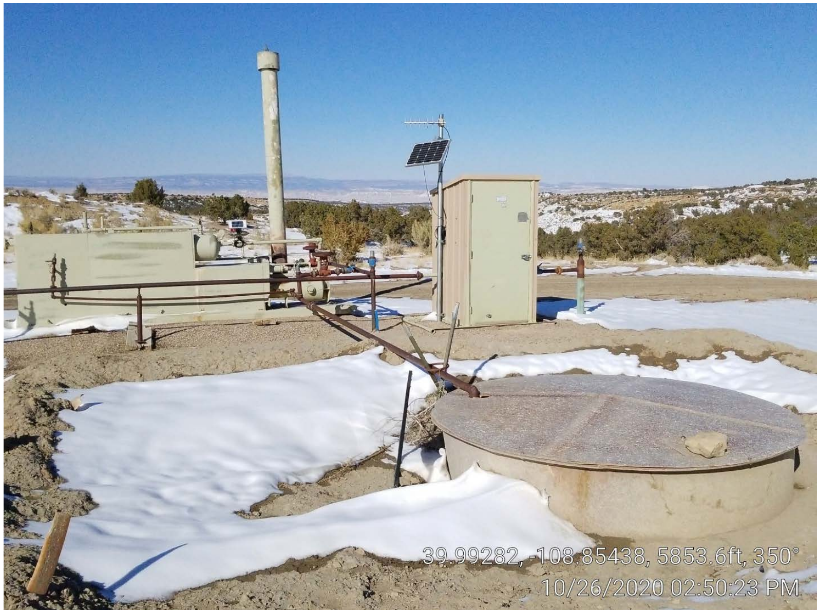
Photo 2. Separator, meter building, tank.
