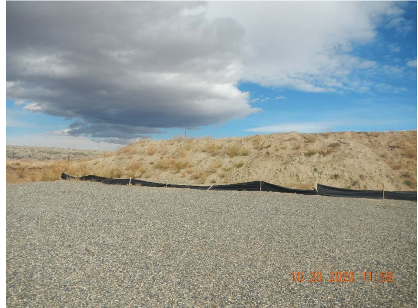
Photo 2. Example of erosion onto location and silt fence becoming debris.
