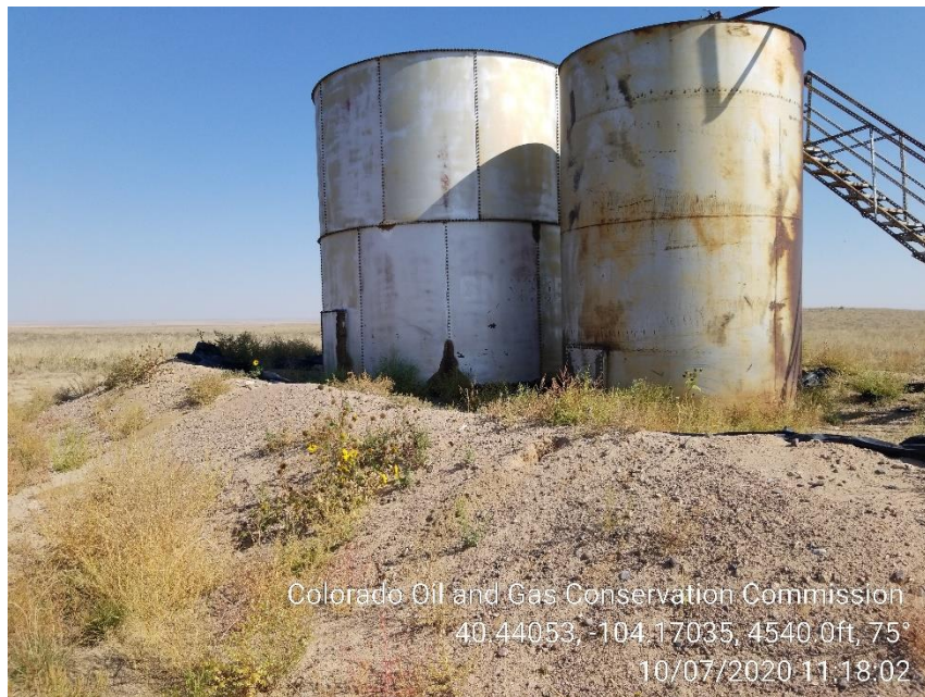
Photo 7 – Tank Battery – Berms Inadequate, Weeds, Rusted Tanks
