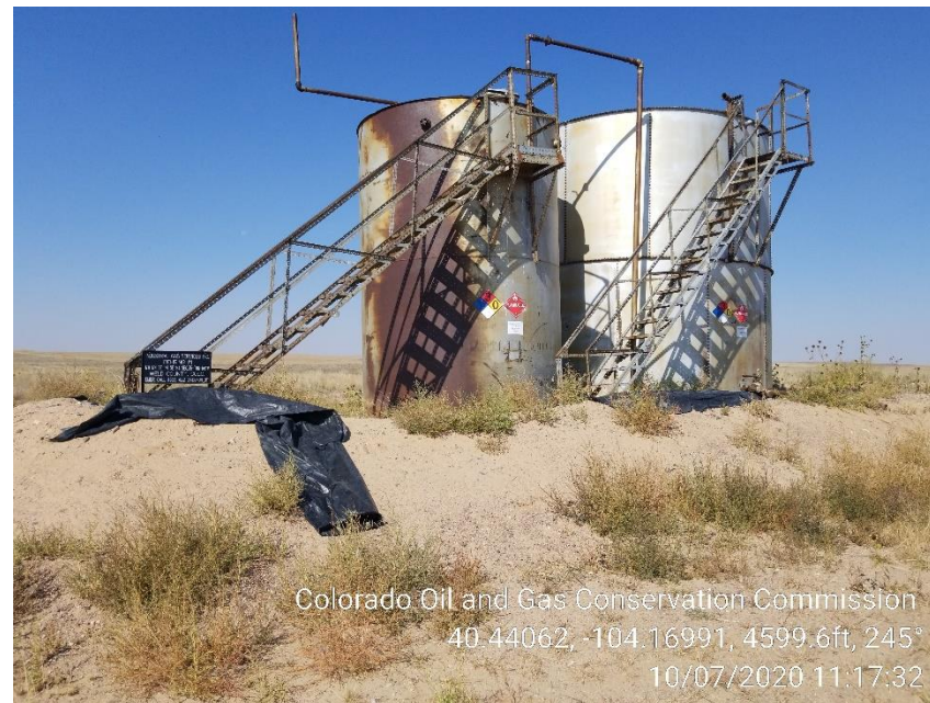
Photo 6 – Tank Battery – Berms Inadequate, Weeds, Rusted Tanks
