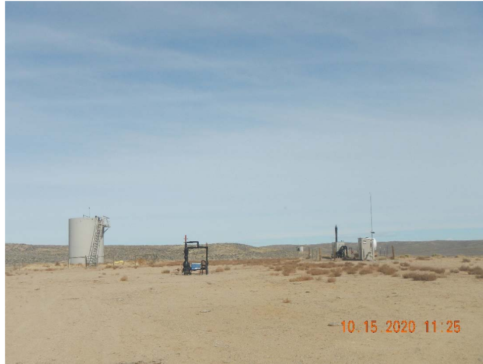
Photo 1. Overview of location taken facing north. Dried annual weeds visible in photo.
