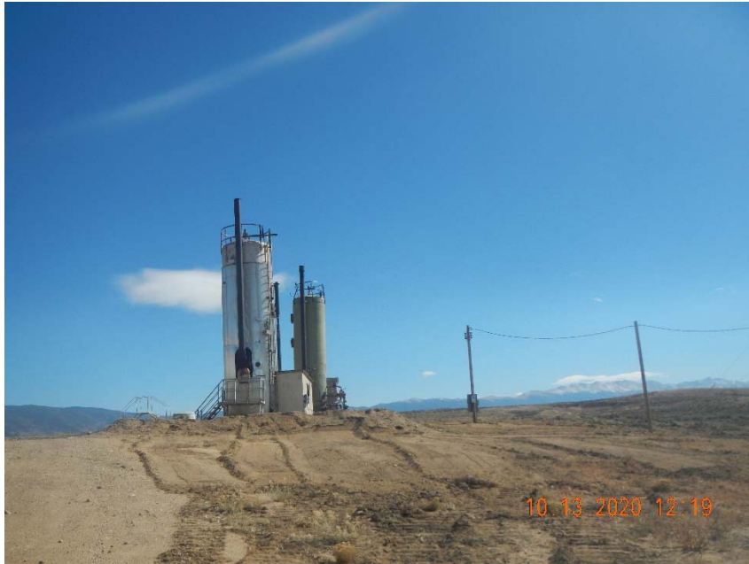
Photo 1. Overview of location taken at entrance facing east. Freshly disturbed soil with no stormwater controls.
