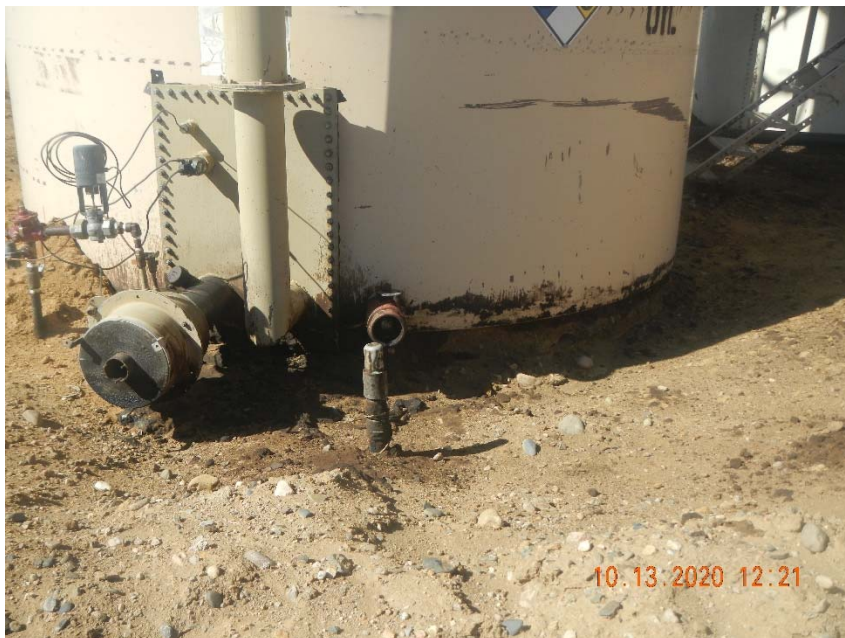
Photo 3. Example of stained soil in tank battery.
