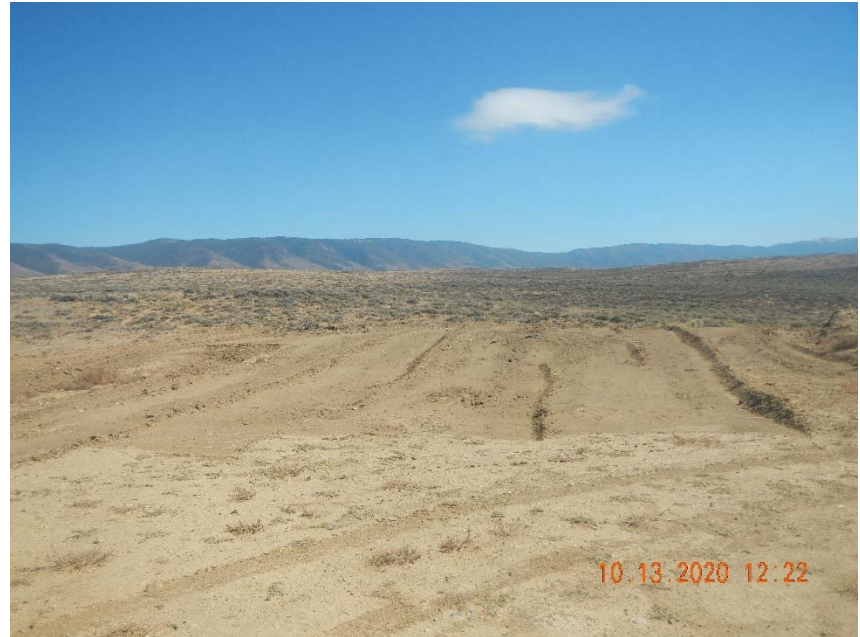
Photo 2. Freshly disturbed soil with no stormwater controls.
