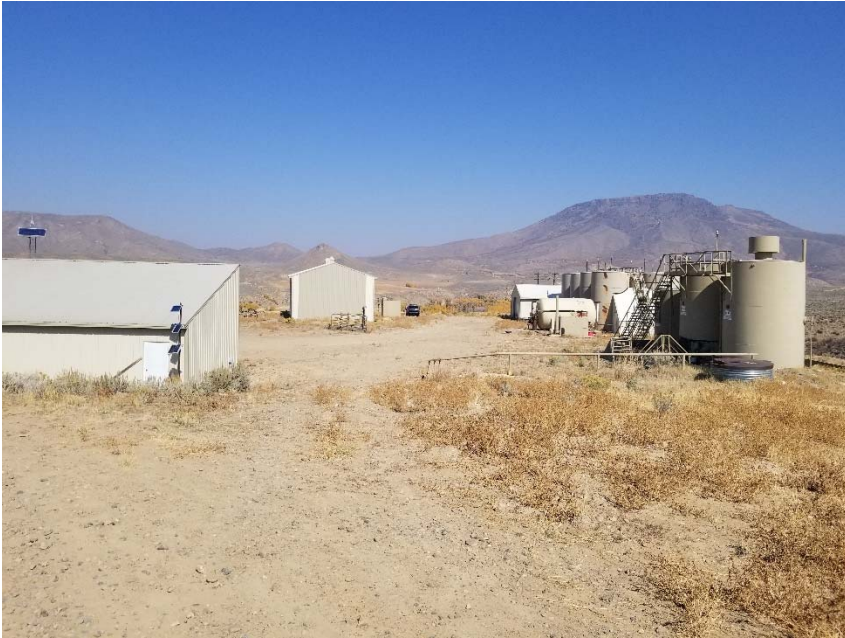
Photo 1. Overview of location taken facing north.
