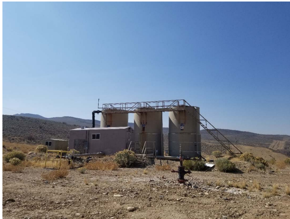
Photo 1. Overview of location taken facing west.
