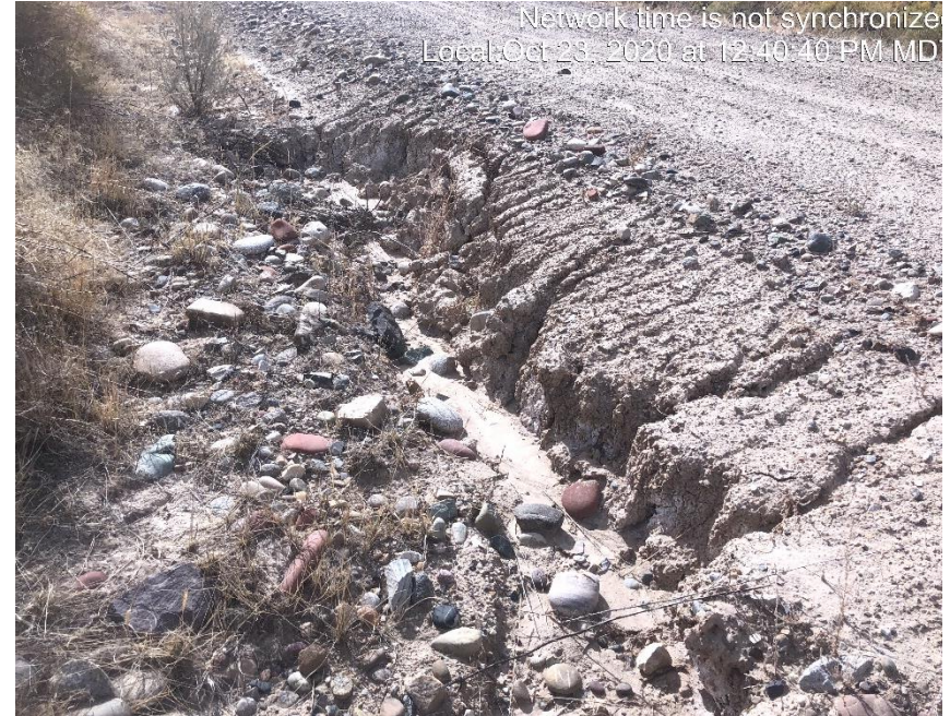
Photo #2105 Multiple places with rill erosion.
