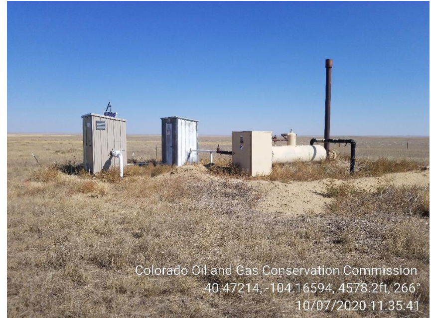
Photo 4 – Separator & Gas Meters – Weeds
