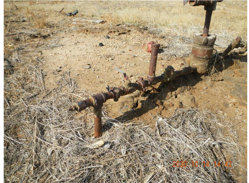
Photo 6: 3" flowline at wellhead.
