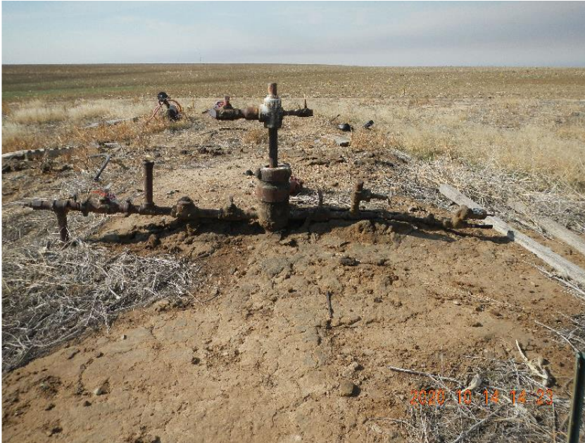
Photo 1: View of wellhead and tree.
