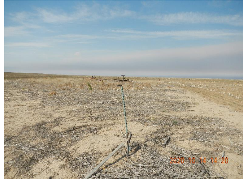
Photo 2: One of three located anchors.
