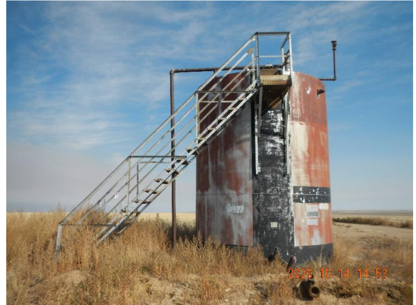
Photo 14: 300 BBL tank at production facility.
