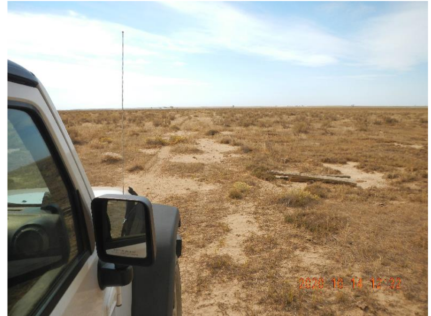
Photo 8: Unmaintained portion of access road.
