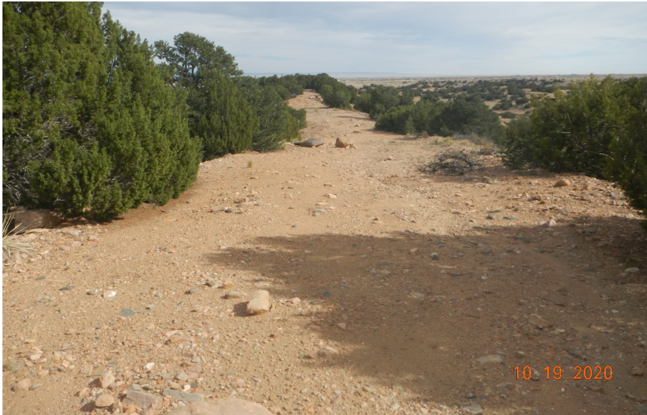
Photo 2. Facing northeast along the access road. The road has not been recontoured and reclaimed. The soils are bare of vegetation and susceptible to erosion.
