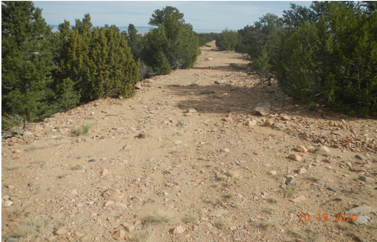
Photo 1. Facing northeast along the access road. The road has not been recontoured and reclaimed. Previous corrective action was not performed.
