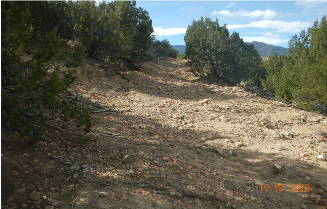
Photo 6. Facing southwest along the access road between the Hassler 24 and Drapper4 well site. This area has not been recontoured and reclaimed and is susceptible to further erosion.
