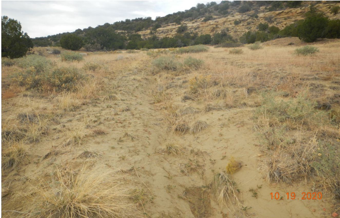
Photo 5. Facing southwest along the former access road. It appears that the stormwater from the location is directed down the road which is causing erosion issues shown in previous photos.
