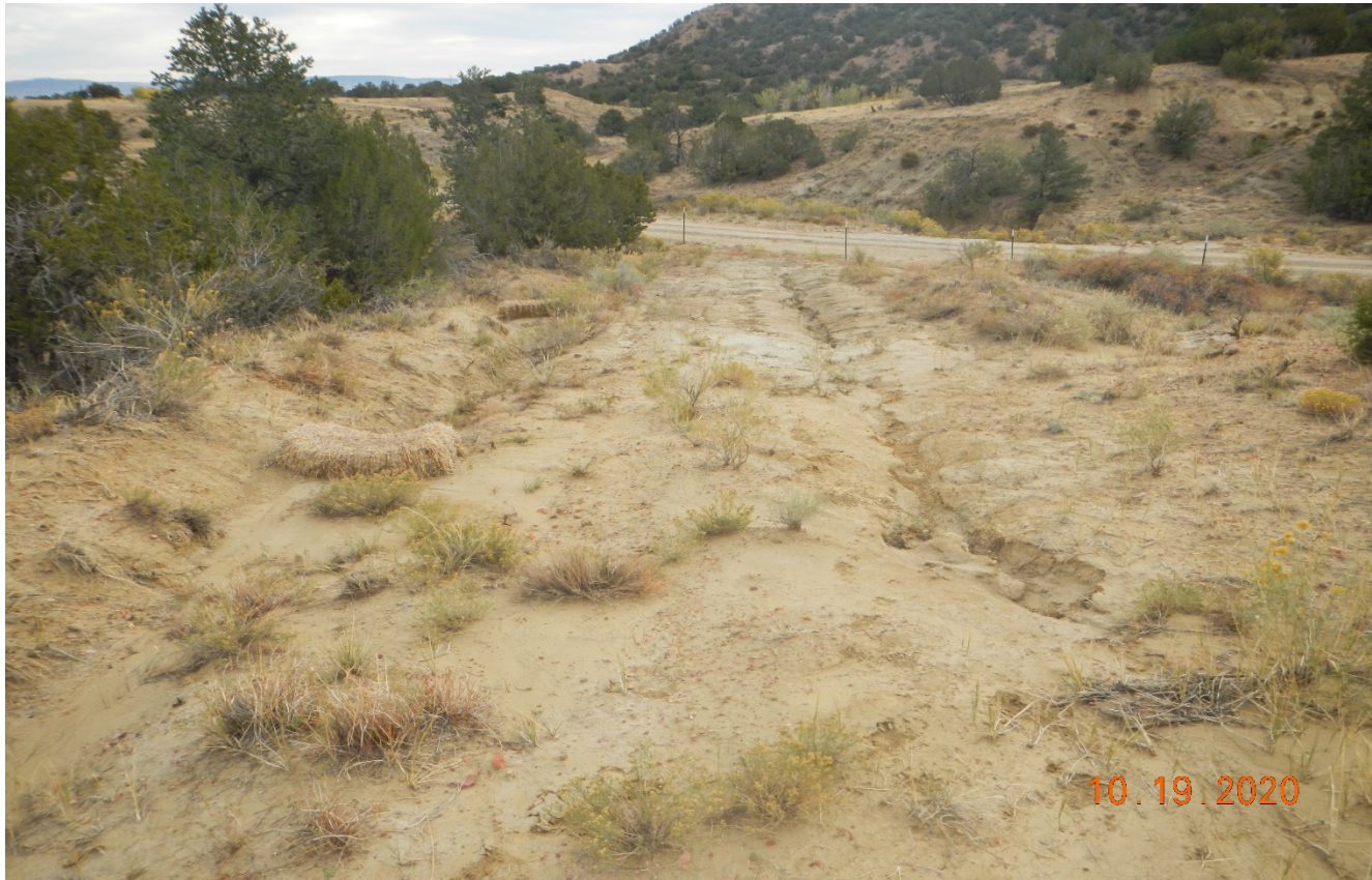
Photo 2. Facing back to the northeast toward the road. There has been straw bales placed along this area however, straw bales are not a long term erosion control and have filled in with sediment. There is an erosion channel directed down toward the main road.
