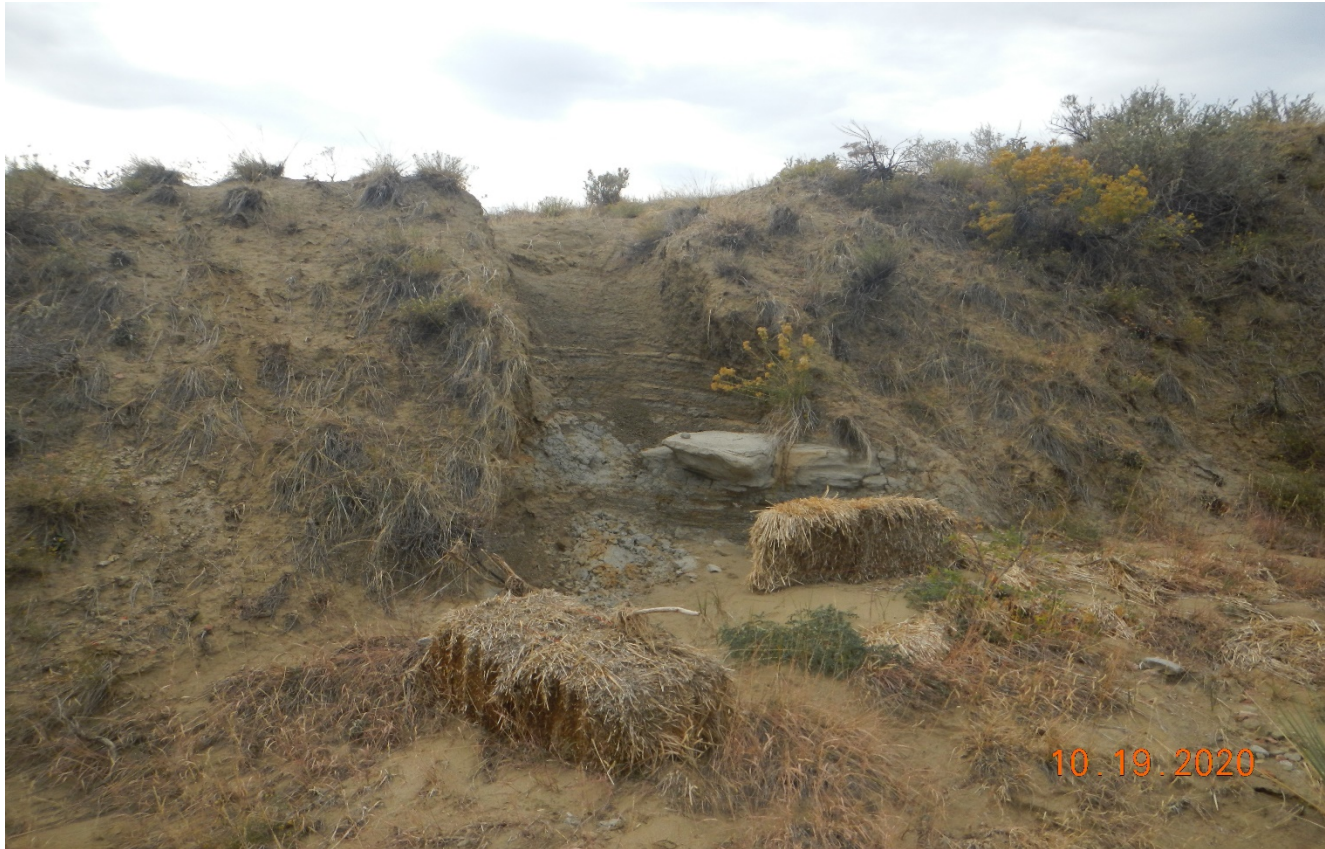
Photo 4. Facing toward the bottom of the erosion shown in previous photo. There is straw bales that appear to have washed out of gully. The gully needs to be filled in and stabilized.
