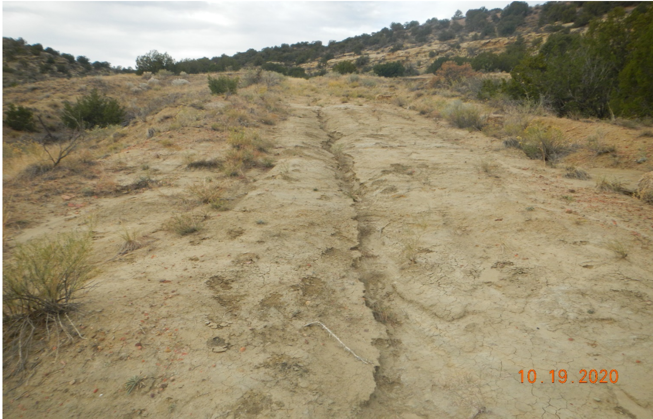
Photo 1. Facing southwest toward the former access road. This area is not stabilized with vegetation and there is erosion occurring.
