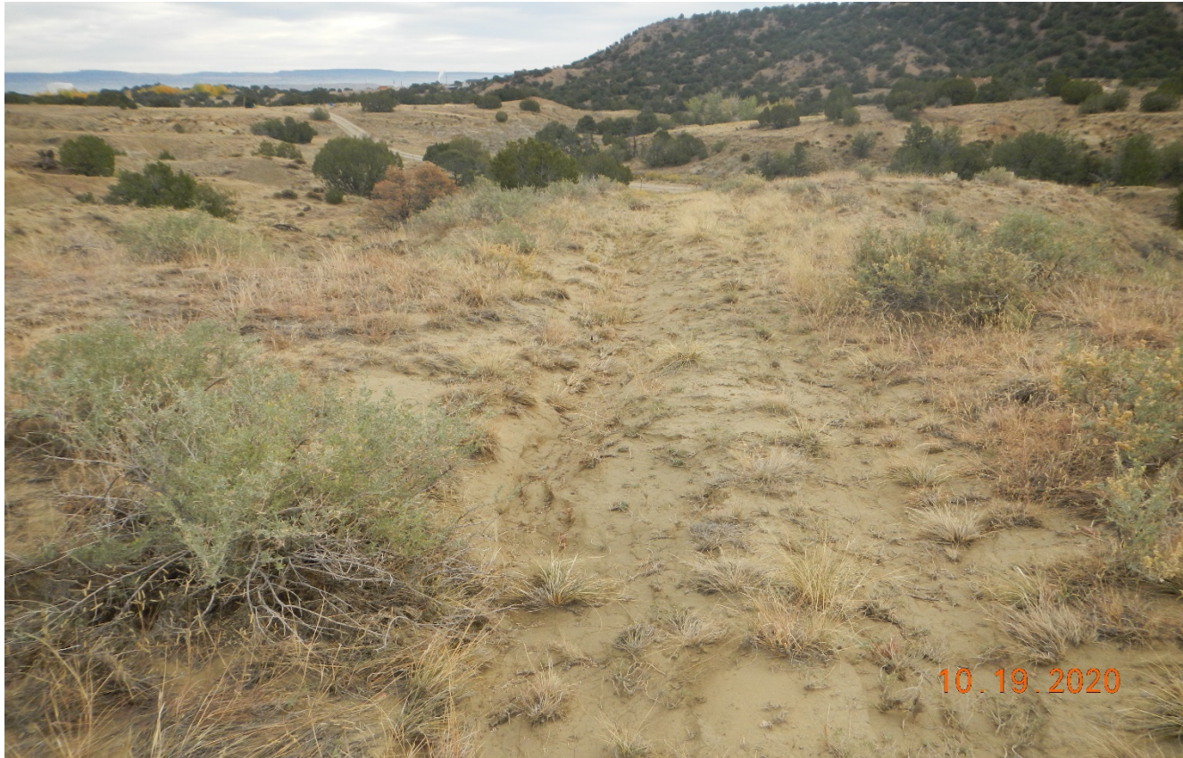
Photo 6. Facing back northeast along the former access road. It appears that the stormwater from the location is directed down the road which is causing erosion issues shown in previous photos.
