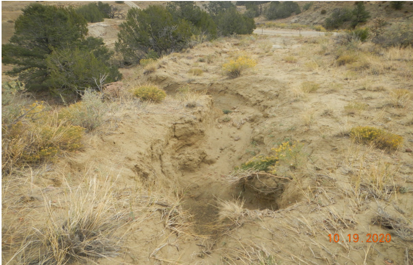
Photo 3. There is an erosion gully along the road that is approximately 2-3 ft. deep. This area needs to be filled in and stabilized. Previous corrective action was not performed.
