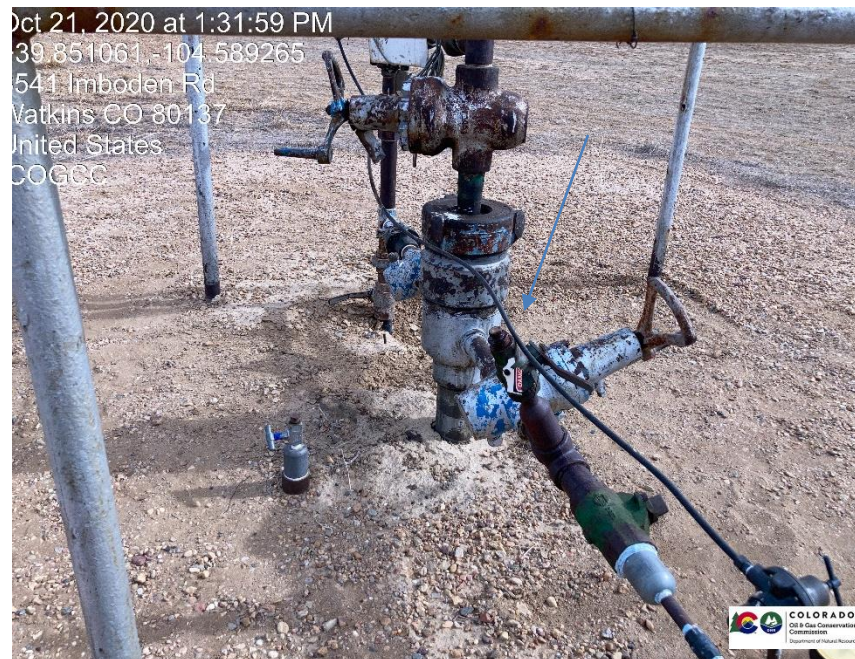
Pic 1 bullplug installed to mitigate leaking valve
