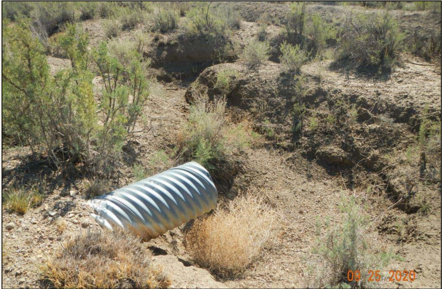
Photo 3. View of another culvert outlet needing stabilization.
