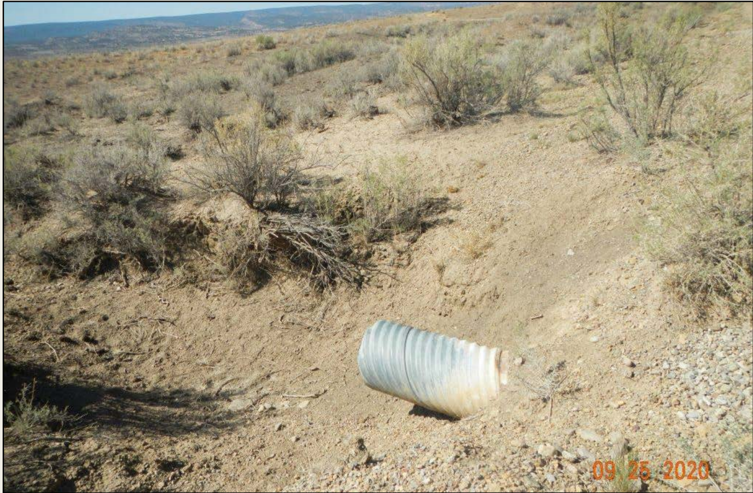
Photo 2. View of culvert outlet along the access road that is not stabilized and above grade.
