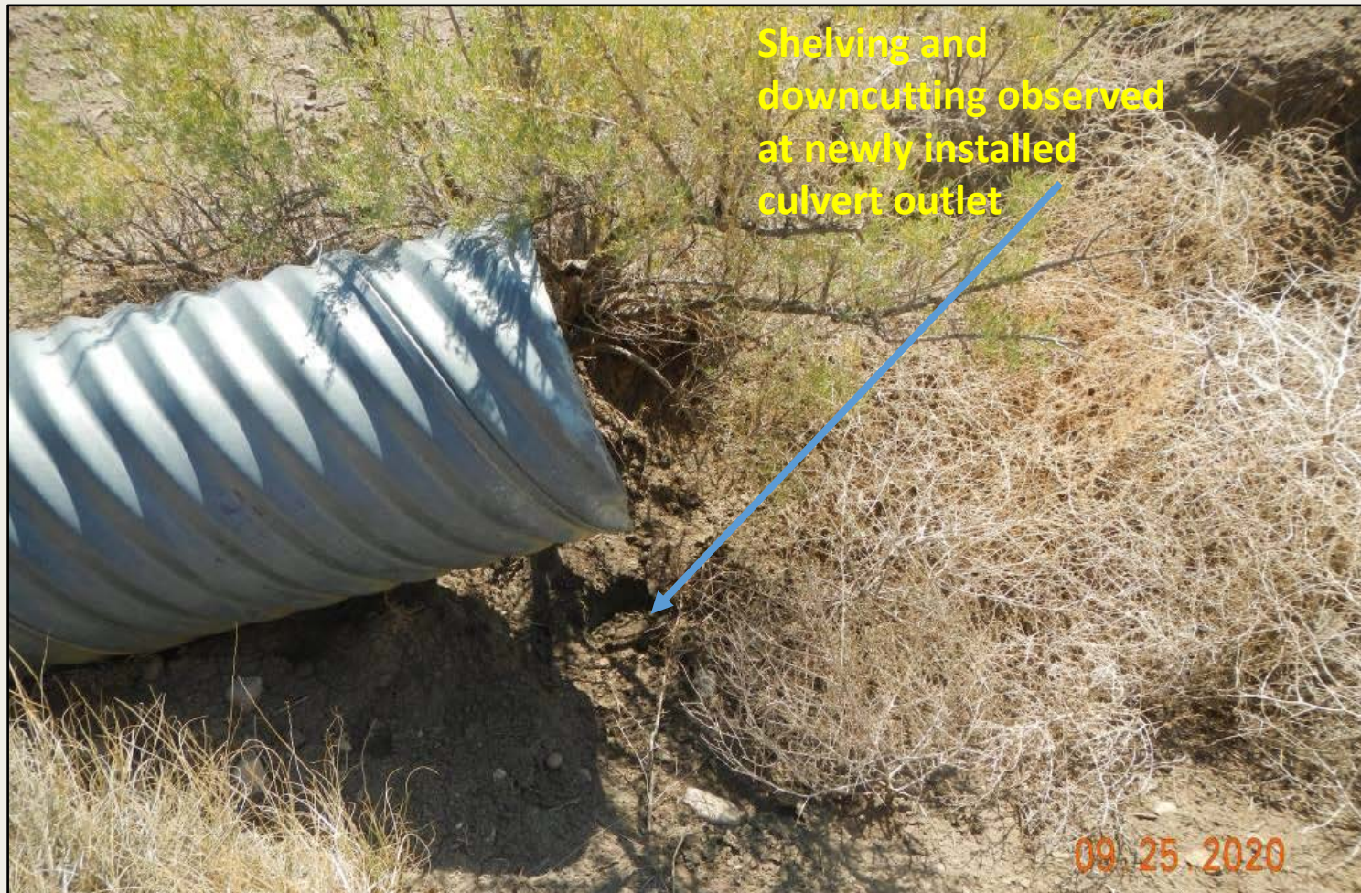
Photo 4. Closeup view of culvert outlet needing stabilization, where you can see erosional down-cutting starting to occur.
