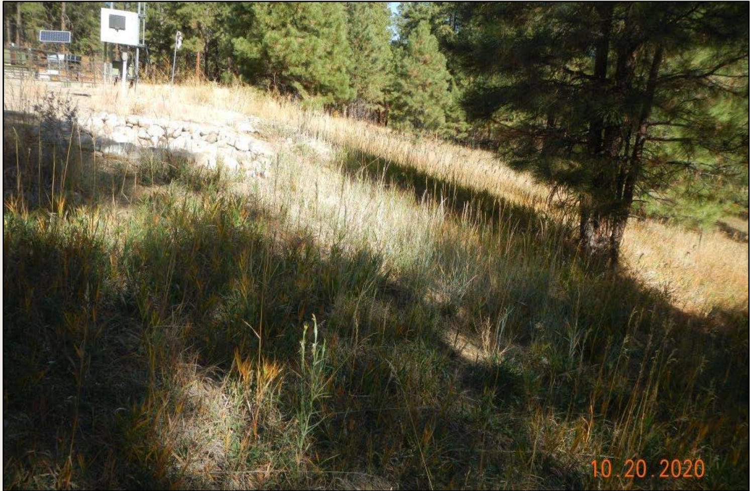
Photo 2. View of the eastern fill slope from the southeastern corner facing northward. Revegetation is progressing with western wheatgrass, sand dropseed, and smooth brome. Stormwater controls appear to be functioning at this time.
