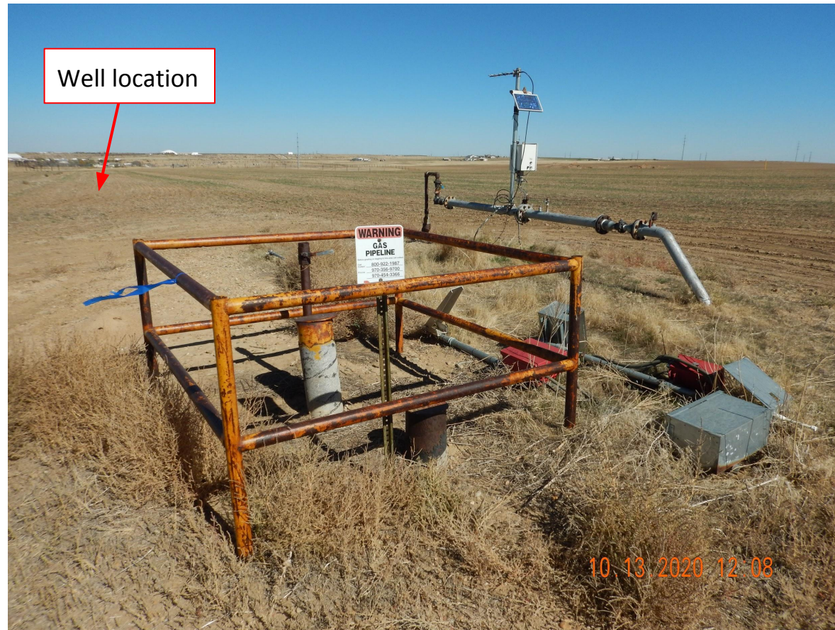
Photo 1. Photo taken from the associated tank battery location, facing North. Photo illustrates the Operator has failed to remove all equipment. DCP was nearby on the day of this inspection and indicated that all equipment was going to be removed.
