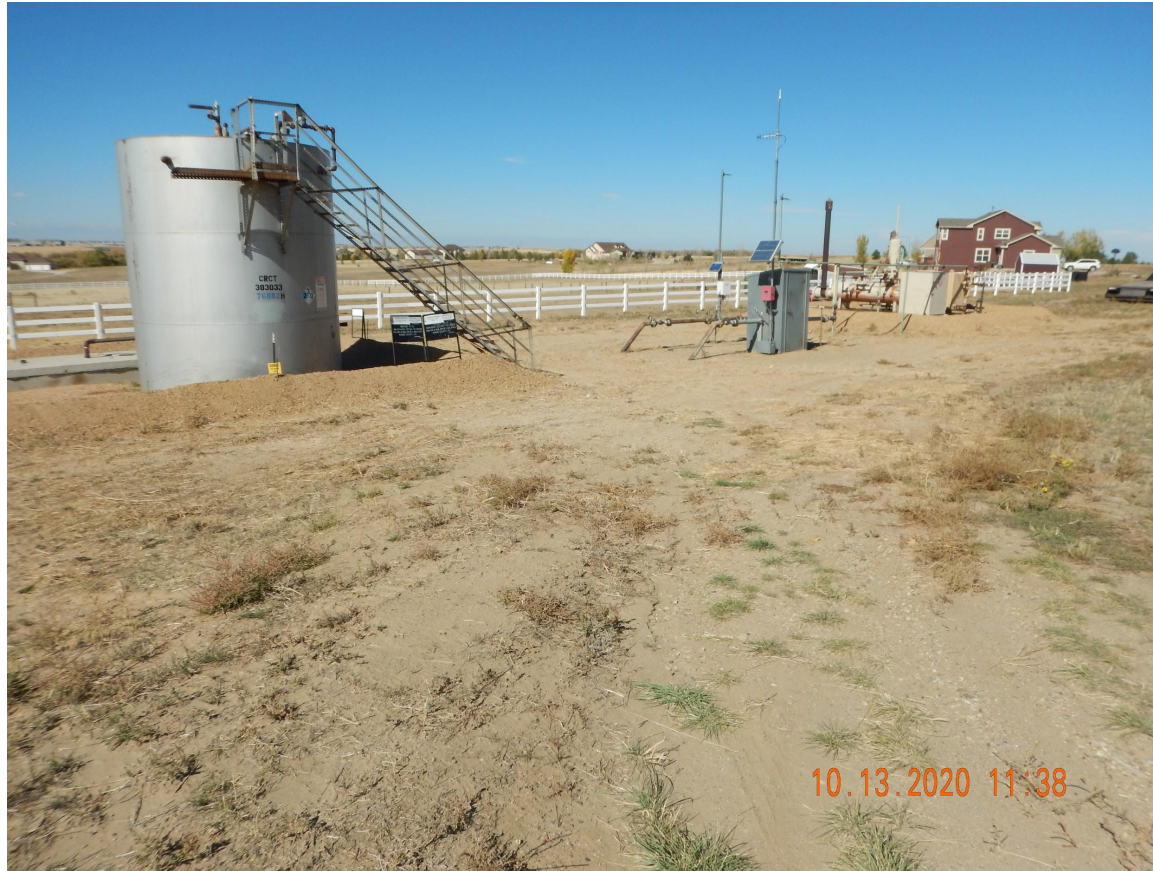
Photo 2. Photo taken from the tank battery, facing North. See comments under Photo 1.
