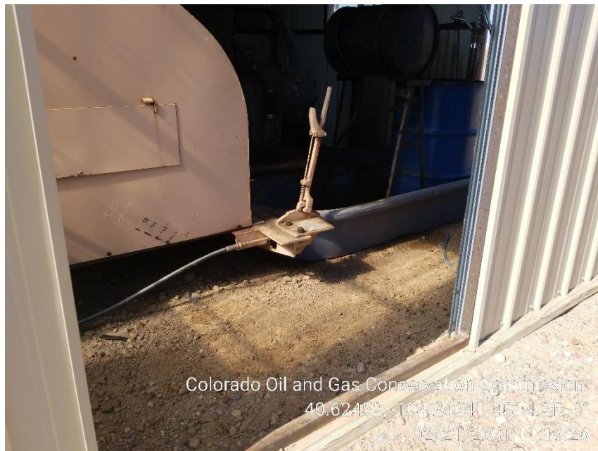
Photo 7 – Stained Soil at Gas Engine
