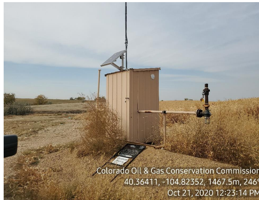
Photo 2: Unused/disconnected gas meter
