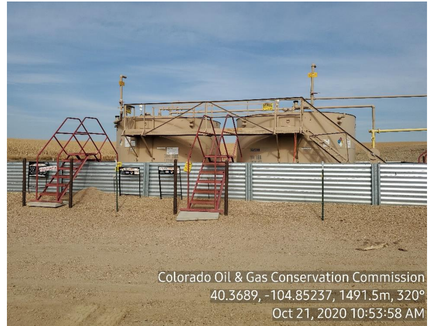
Photo 2: Tank Battery
