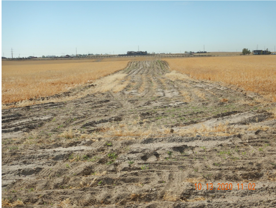
Photo 1. Photo taken from the entrance of the well location off 132nd Ave, facing South. Photo illustrates Operator has removed equipment from the well location and has removed gravel from the well location and access road, and has performed seedbed prep.
