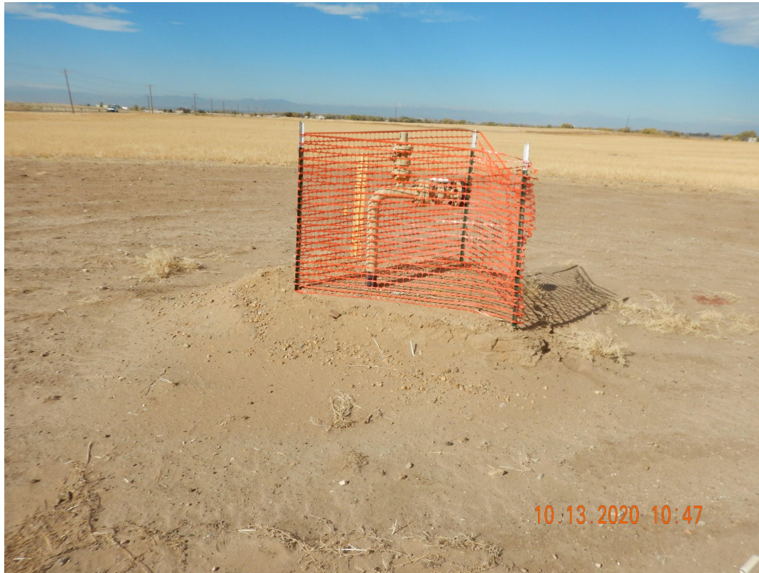
Photo 3. Photo taken from the associated offsite tank battery, facing West. Photo illustrates Operator has failed removed all equipment related to the PA well.
