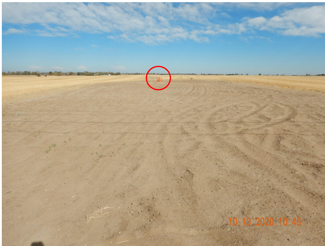
Photo 1. Photo taken from the entrance of the associated offsite tank battery, as well as the PA well location off 128th Ave, facing North. Photo illustrates Operator has failed removed all equipment related to the PA well. Operator has removed gravel from the tank battery, well location and access road, and has performed seedbed prep.
