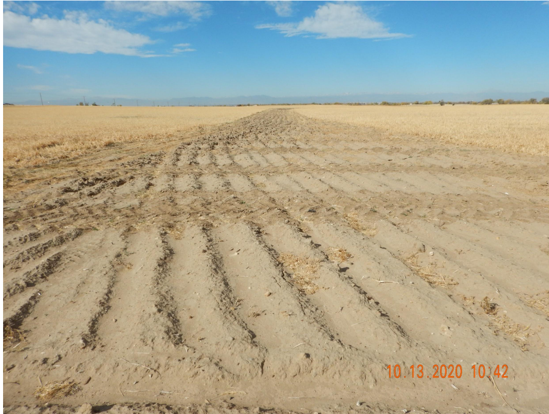
Photo 1. Photo taken from the entrance of the PA well location off Picadilly Rd, facing West. Photo illustrates Operator has removed all equipment related to the PA well, removed gravel and has performed seedbed prep.
