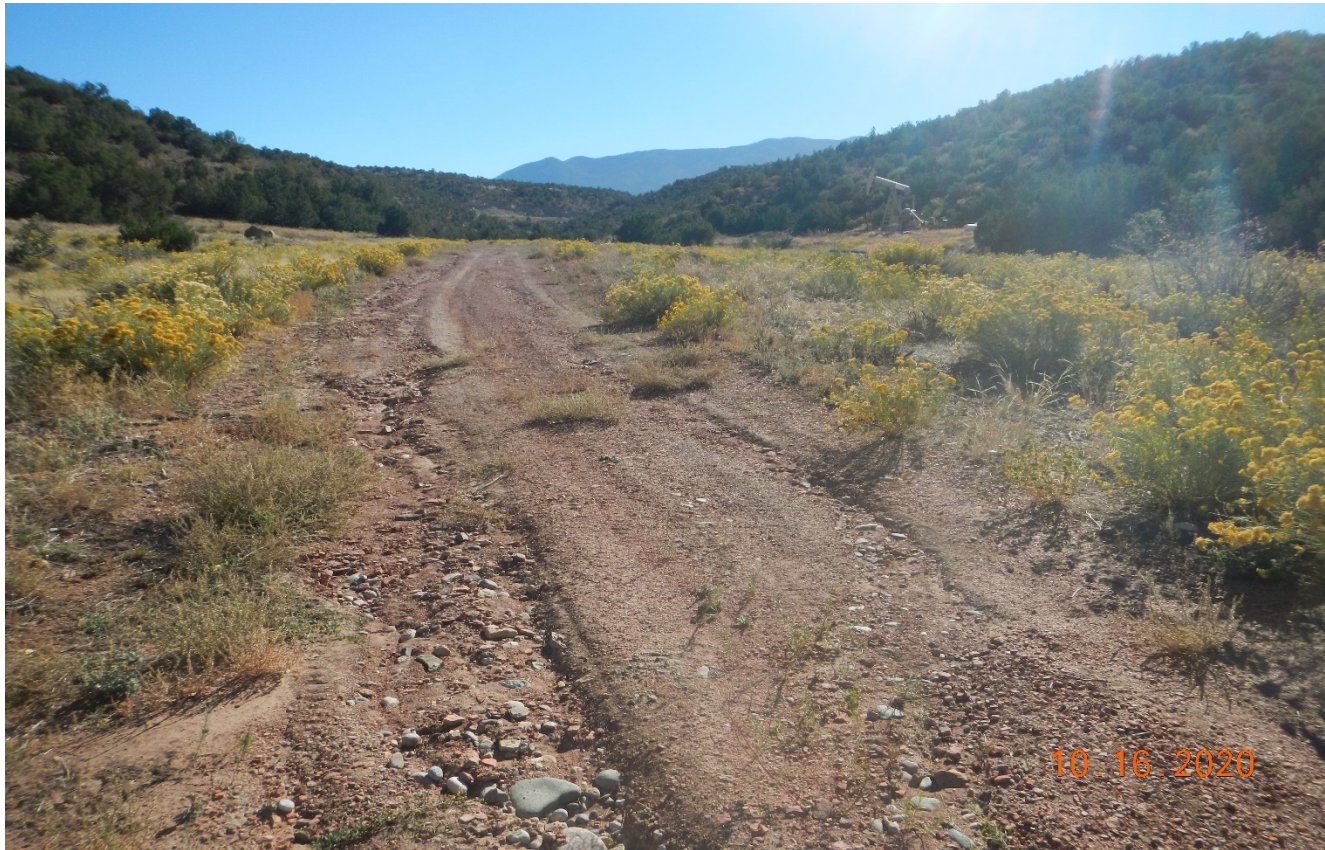
Photo 1. Facing south along the access road. There is erosion occurring down the road which needs to be repaired and stormwater needs to be diverted off the road.
