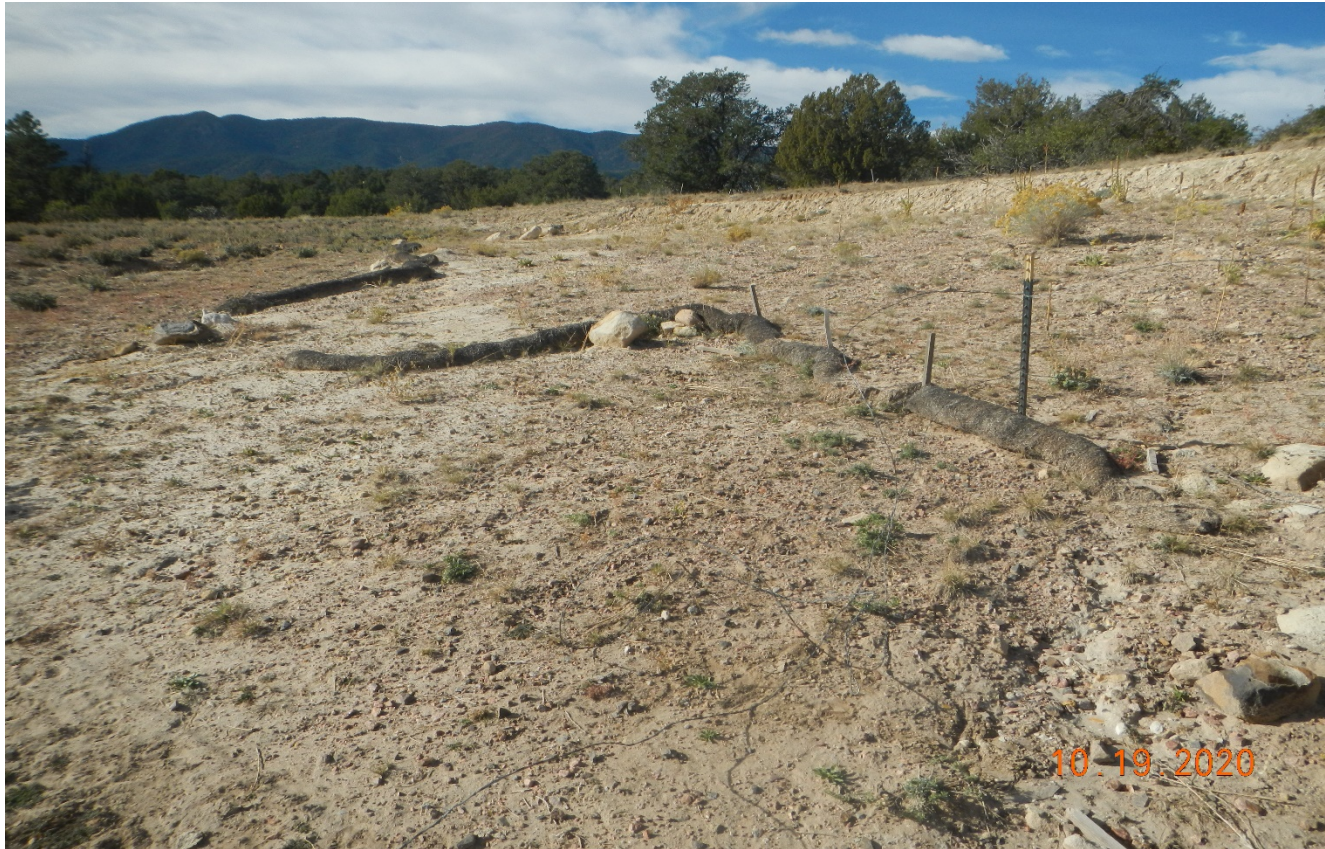
Photo 5. There are wattles displaced at the southwest side of the location. This was also observed in the previous inspection. Wattles need to be repired and maintained.
