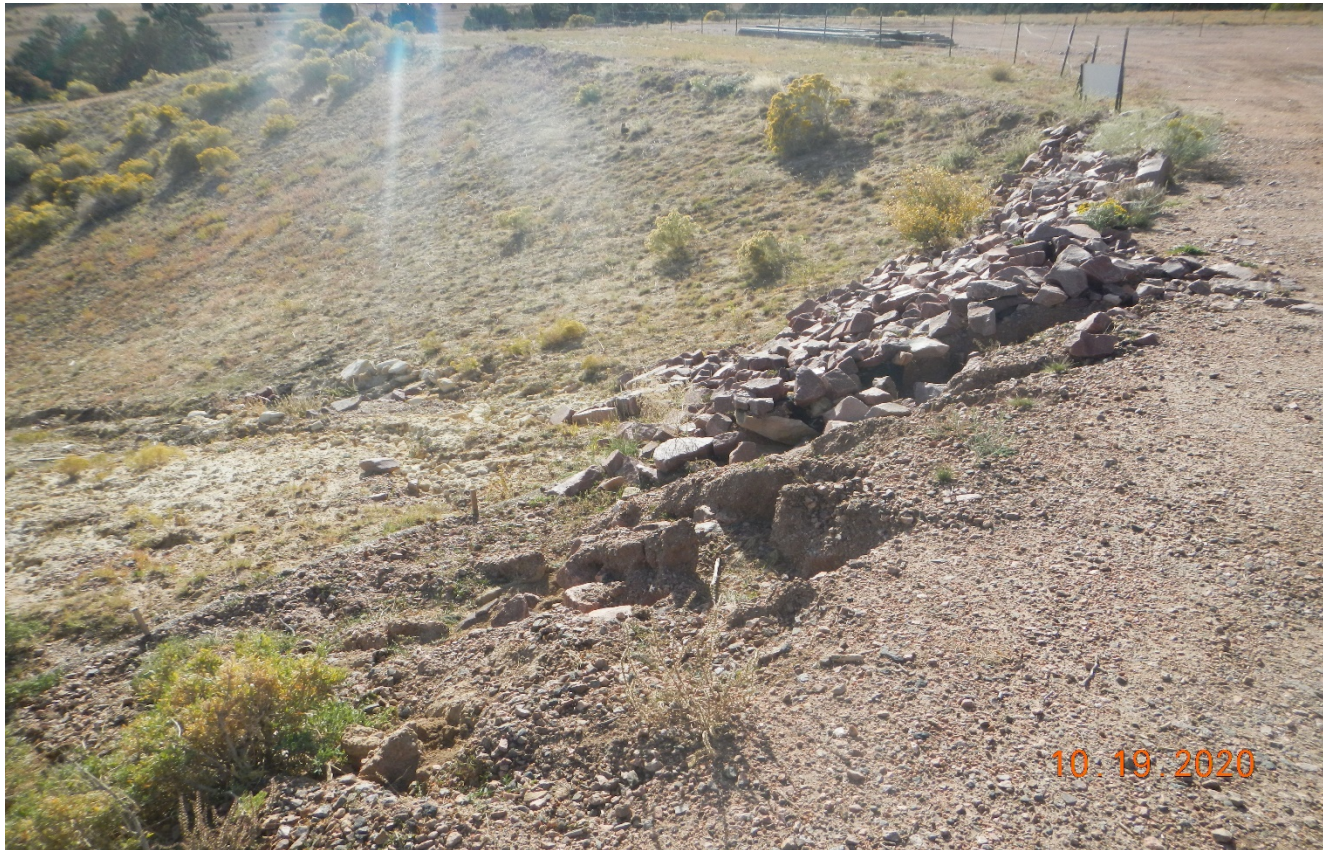
Photo 9. There is erosion occurring across the road at the north side of the location caused by stormwater directed from the top perimeter ditch shown in the previous photo.
