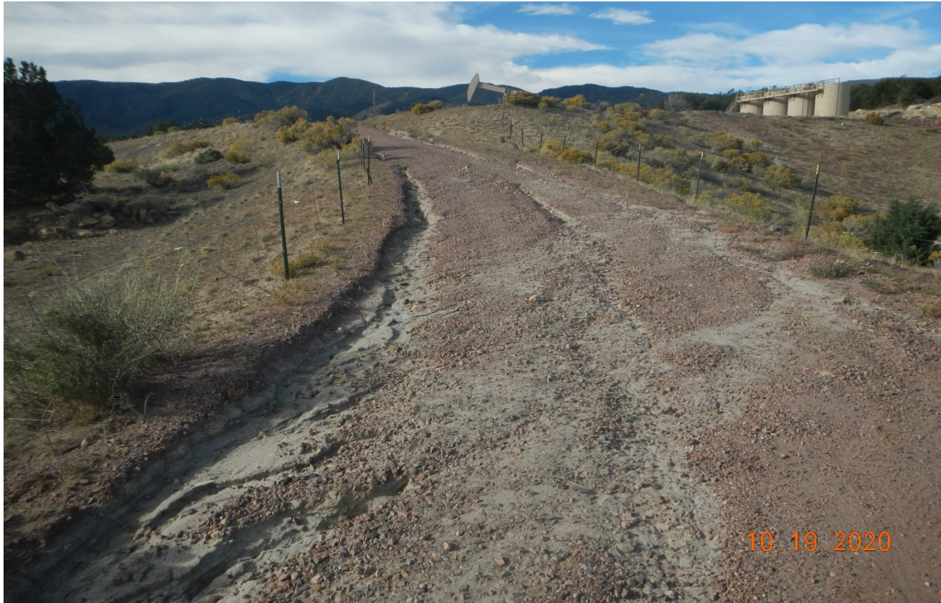
Photo 2. There is erosion along the access road. Stormwater is diverted down the road and into drainage area shown in previous photo. The erosion needs to be repaired and stormwater needs to be properly diverted.
