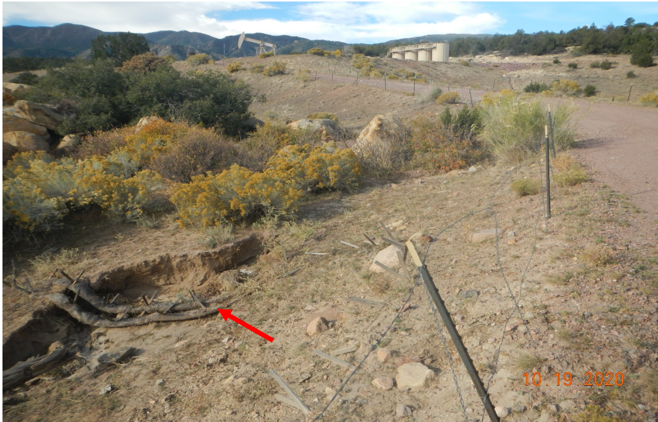
Photo 1. Facing southwest along the access road. Stormwater from the road is creating erosion in area shown at red arrow.. The wattles placed in this area are displaced and are not controlling erosion.
