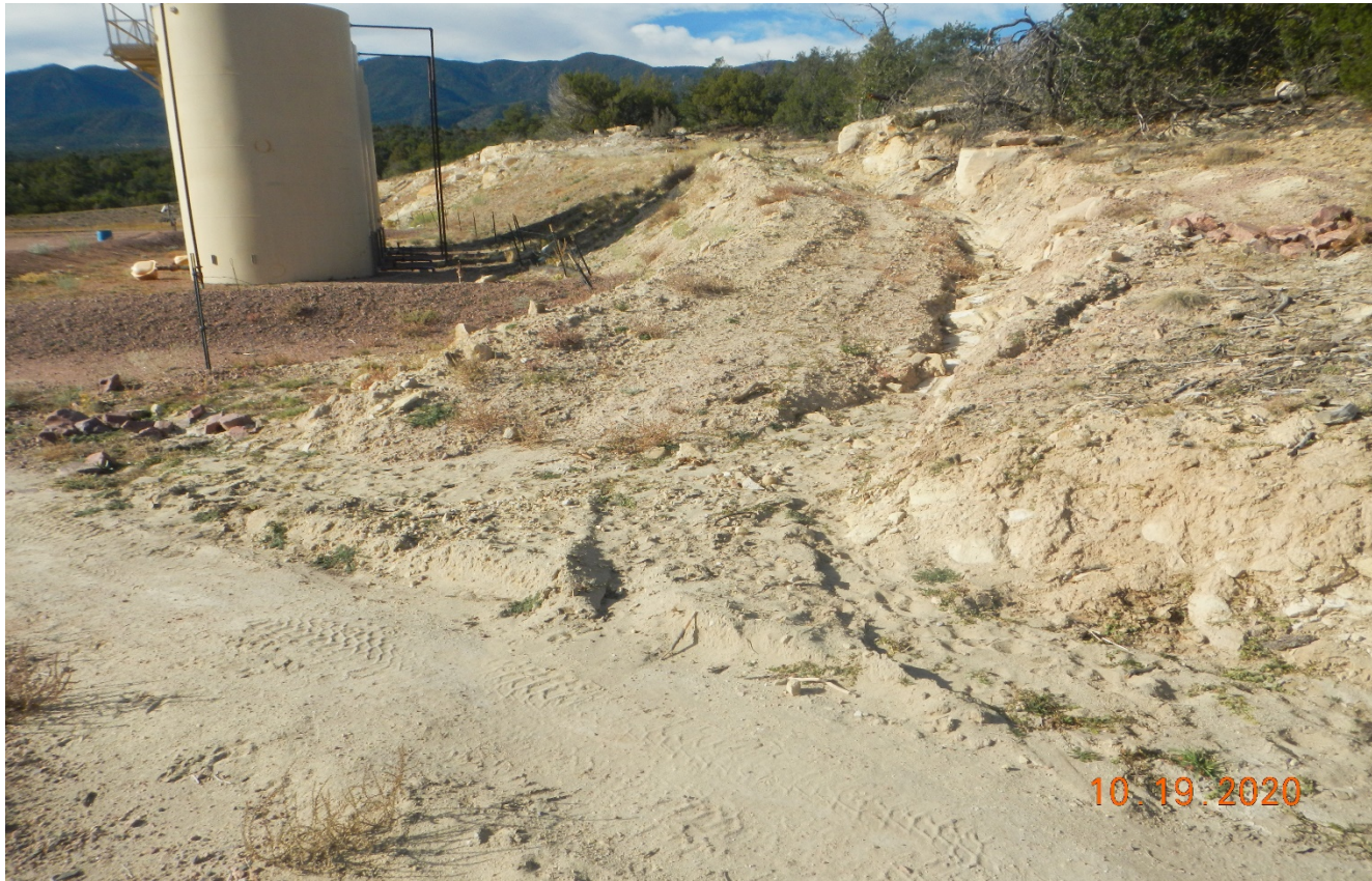
Photo 8. The top perimeter ditch is directing stormwater toward the road which has deposited sediment onto the road. BMP's are needed in this area.
