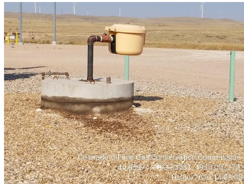
Photos 6 – Stained Soil at Compressor Drain Pit
