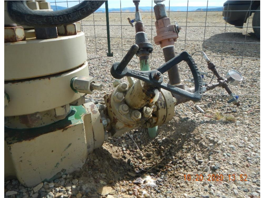
Fluid leaking from wheel valve on annulus.
