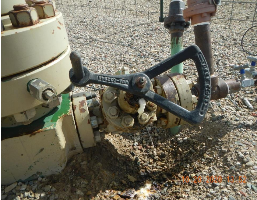
Fluid leaking from wheel valve on annulus.
