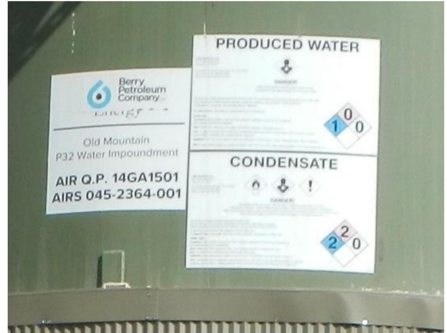
**No phone number and tank capacity on tank.**
