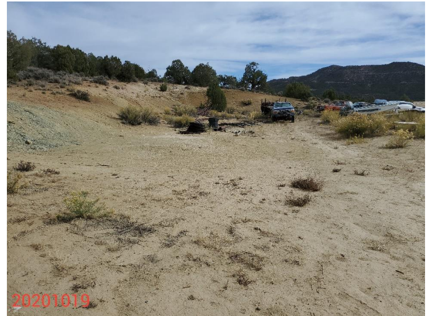
Photo 4: Photo taken from the north end of the Location, facing east. Photo shows areas documented in previous inspection that were required to be reclaimed pursuant to 1003 interim reclamation requirements. Photo shows unused equipment, equipment not needed for production, or trash debris remains, and that interim reclamation activities (including but not limited to recontouring/regrading, compaction alleviation, revegetation) have not been conducted per 1003 rules.
