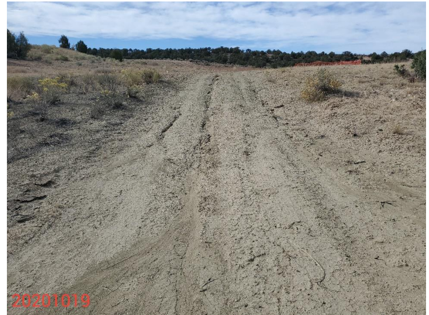
Photo 2: Photo taken from the east end of the Location, facing southwest. Photo shows access road through the Location has not been reclaimed.
