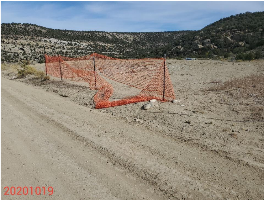
Photo 1: Photo taken from the west end of the Location, facing northeast. Photo shows fence has been installed to prevent access to road traveling through Location. Access road through Location has not been reclaimed in accordance with COGCC 1004 rules.
