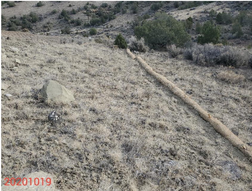
Photo 3: Photo shows example of wattles installed along perimeter of Location and access road.
