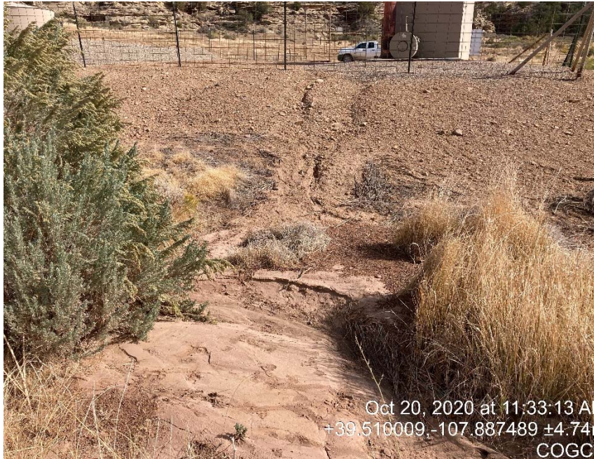
BMP's need maintenance / Run off of sediment
