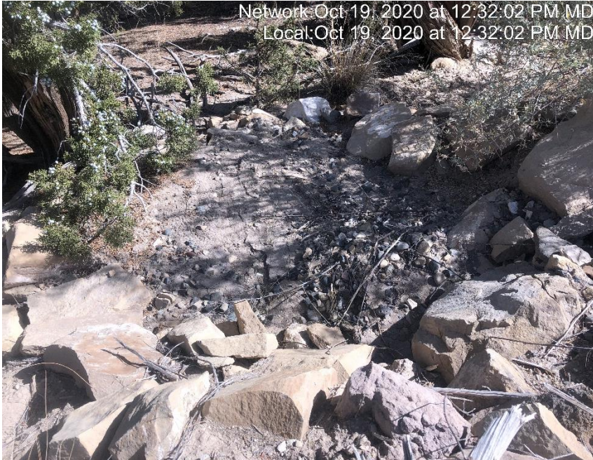
Photo #2046 Sediment trap is full.
