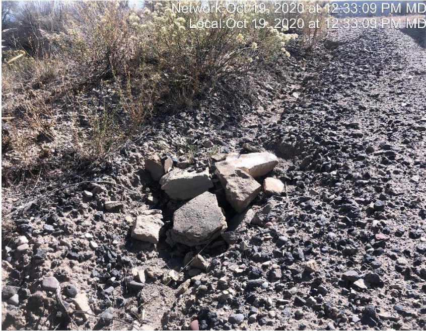
Photo #2048 Rill erosion around check dam.
