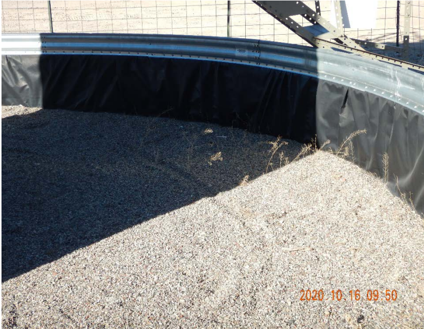
Photo #5 – Vegetation growth inside of secondary containment area.
