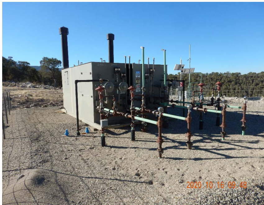
Photo #3 – Heated horizontal separators on south end of pad.
