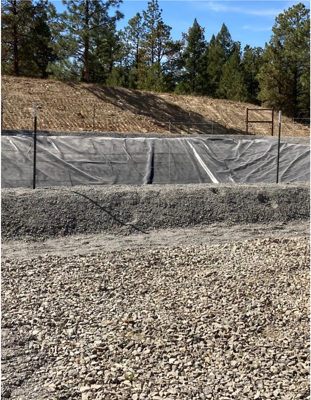
Replaced compromised Pit Liner per Rule 904
