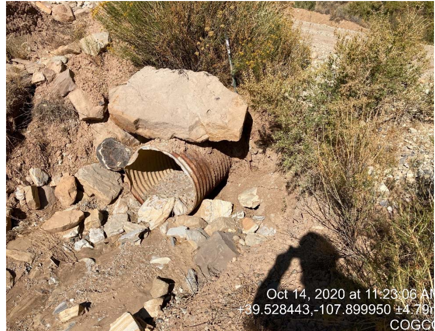
South side of road at entrance to location sediment coming through culvert.
