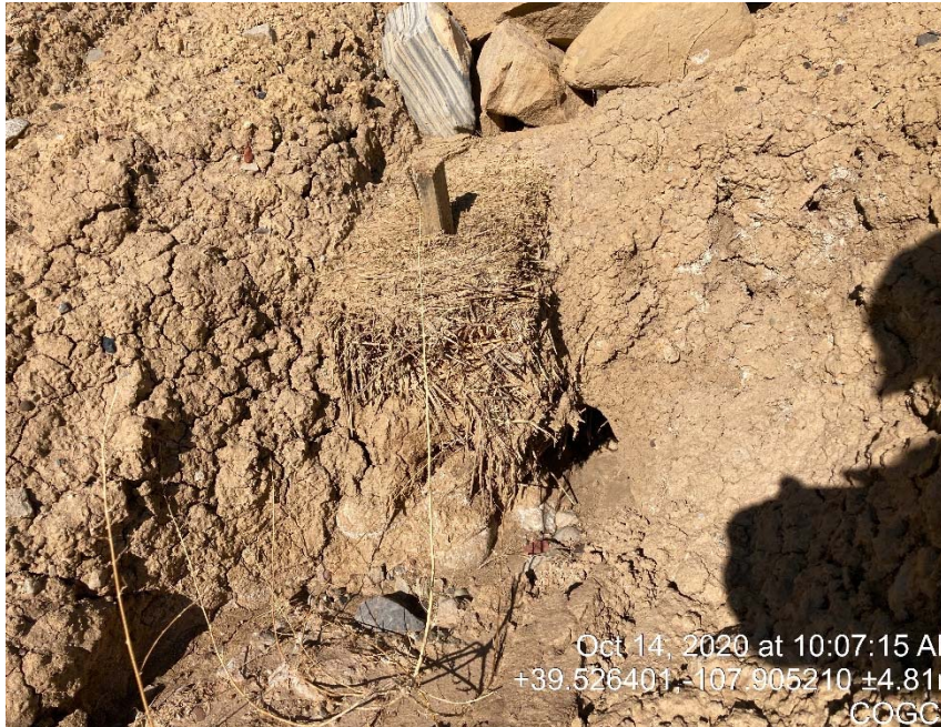
Erosion undercutting of BMP's
