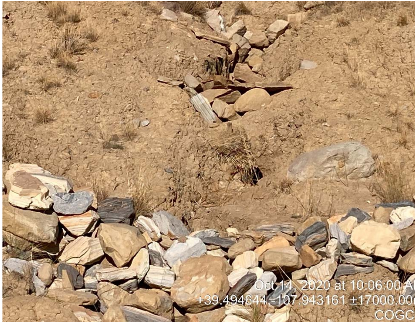
Erosion undercutting of BMP's
