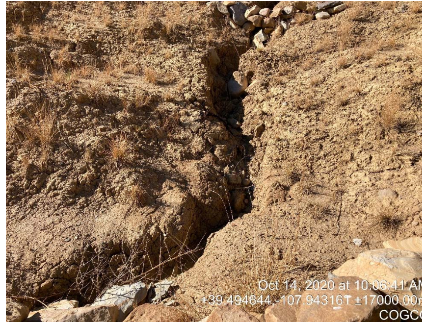
Erosion undercutting of BMP's
