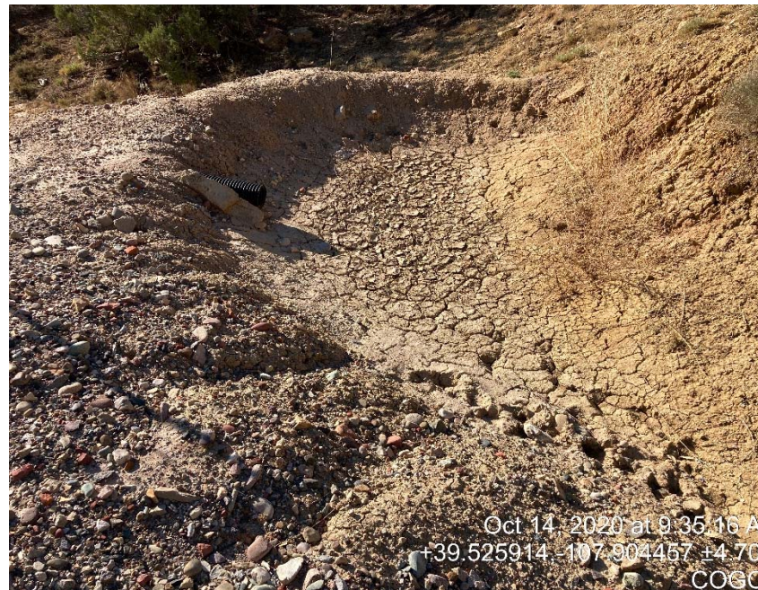
Sediment trap with drain
