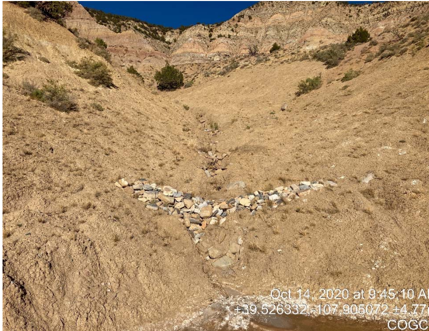
Erosion undercutting of BMP's
