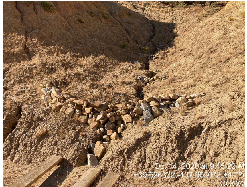
Riling and Erosion undercutting of BMP's
