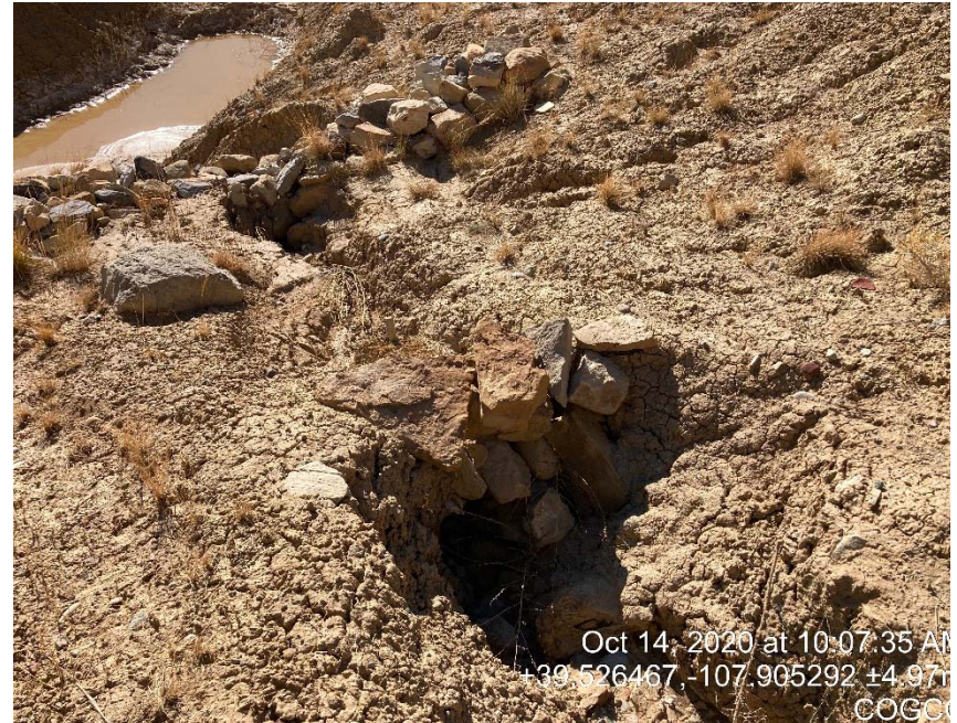
Erosion undercutting of BMP's
