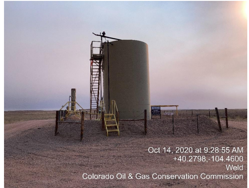
Photo #2 Tank Battery
