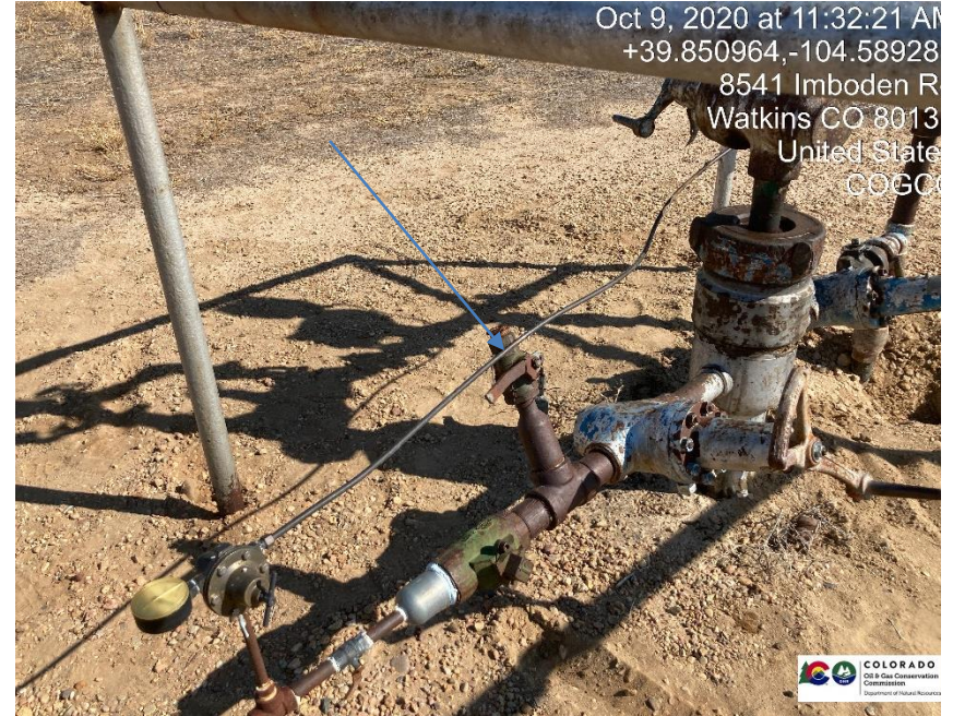
Pic 2 mechanical issue on valve on casing line venting gas
