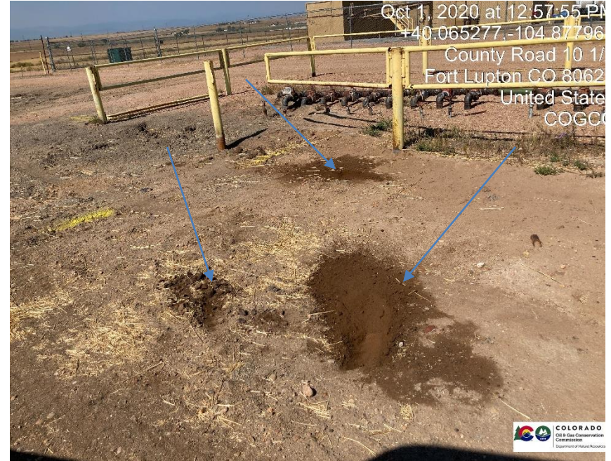
Pic 2 stained soil where flow lines come into manifold
