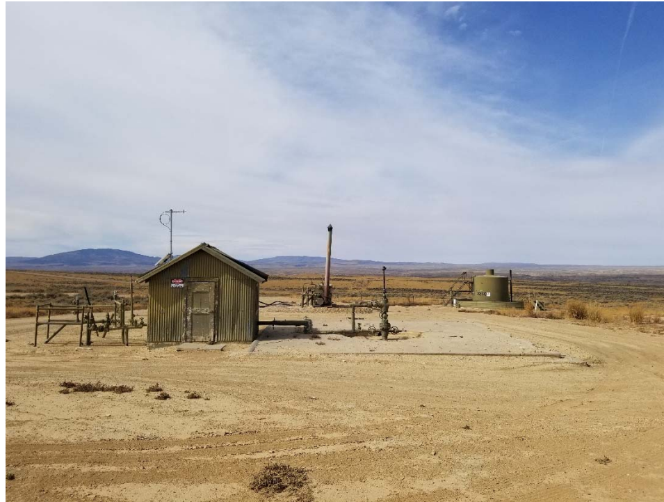
Photo 1. Overview of location taken facing north.
