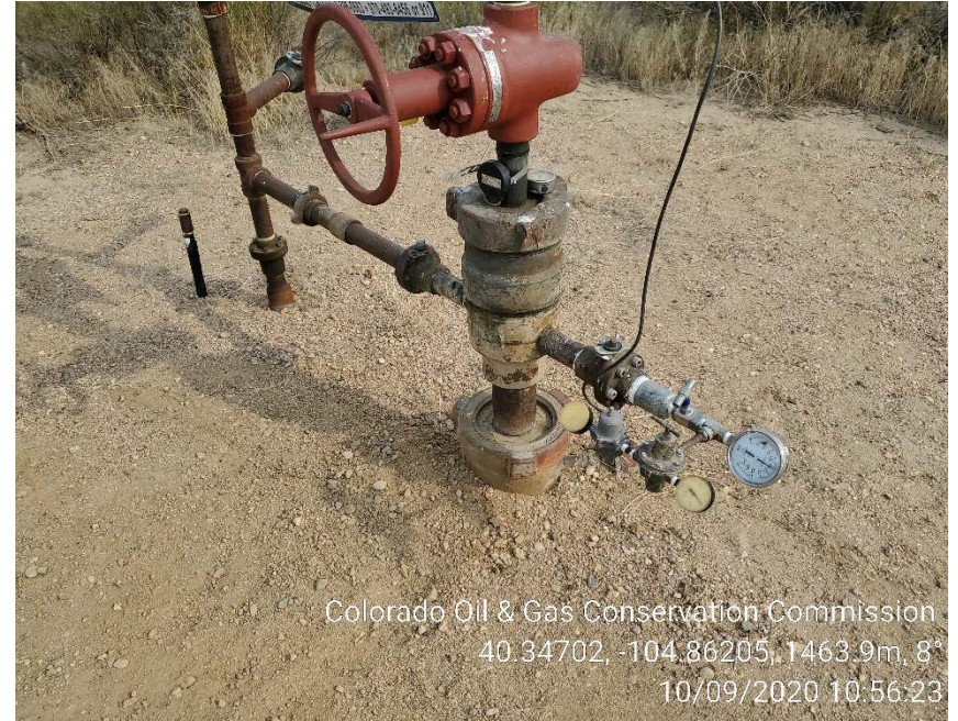
Master valve leak and stained soil on 10/9/2020
