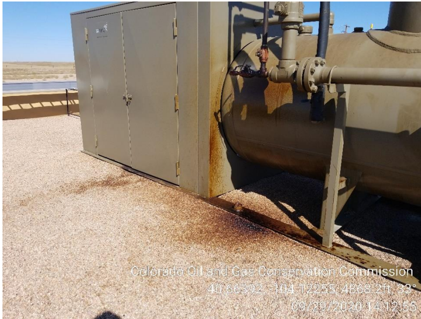
Photo 7 – Stained Soil at West Separator
