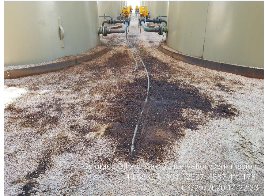
Photos 19 – Stained Soil at Tanks
