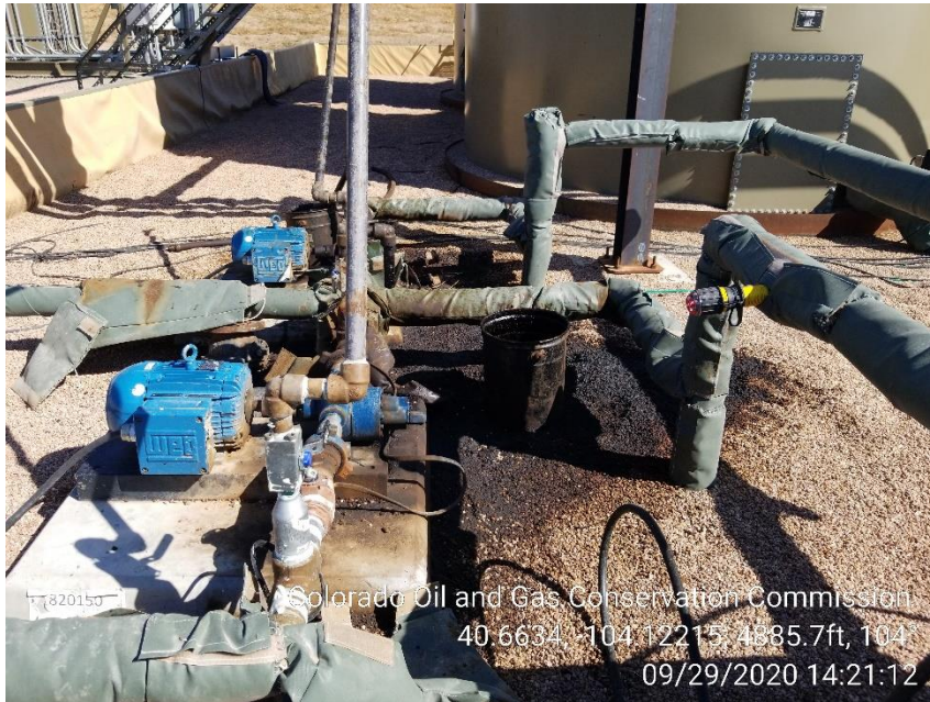
Photo 17 – Stained Soil at the Recycle Pump
