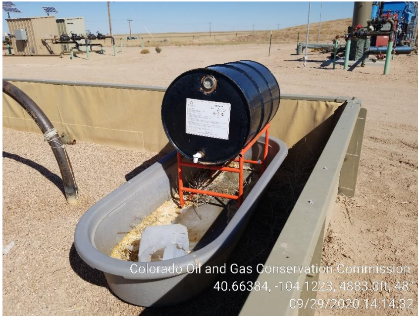
Photo 5 – Secondary Containment needs Wildlife Netting
