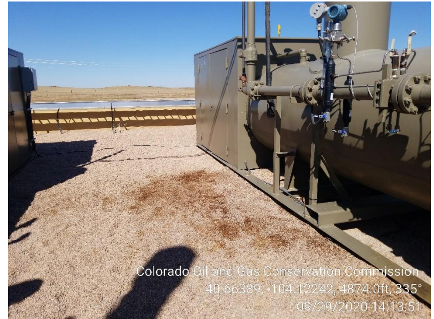
Photo 8 – Stained Soil at Middle Separator
