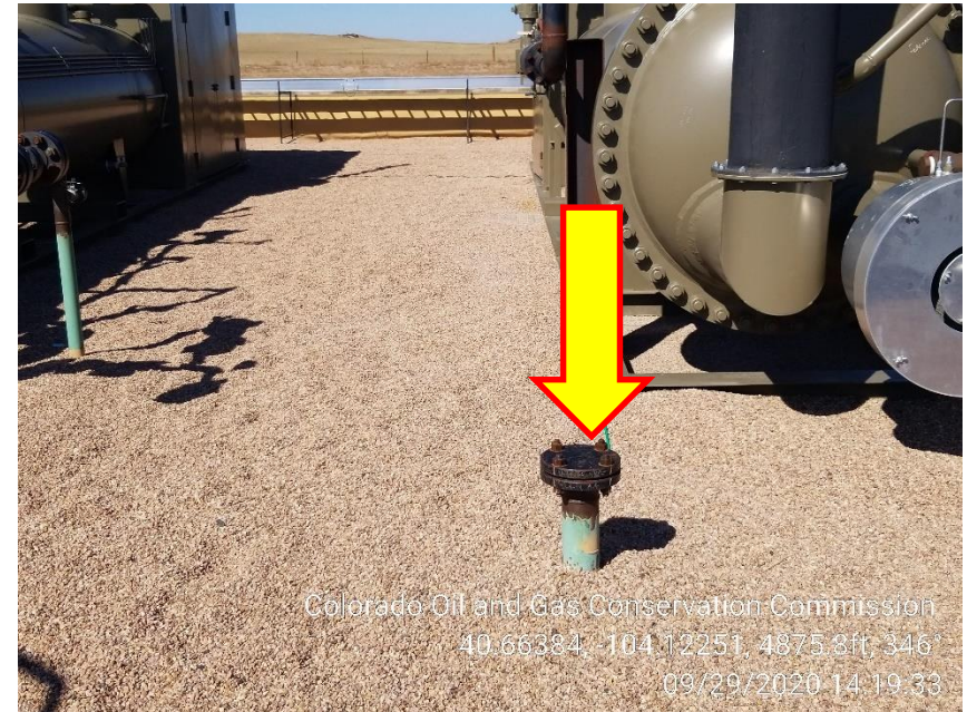
Photo 6 – Unmarked Riser
