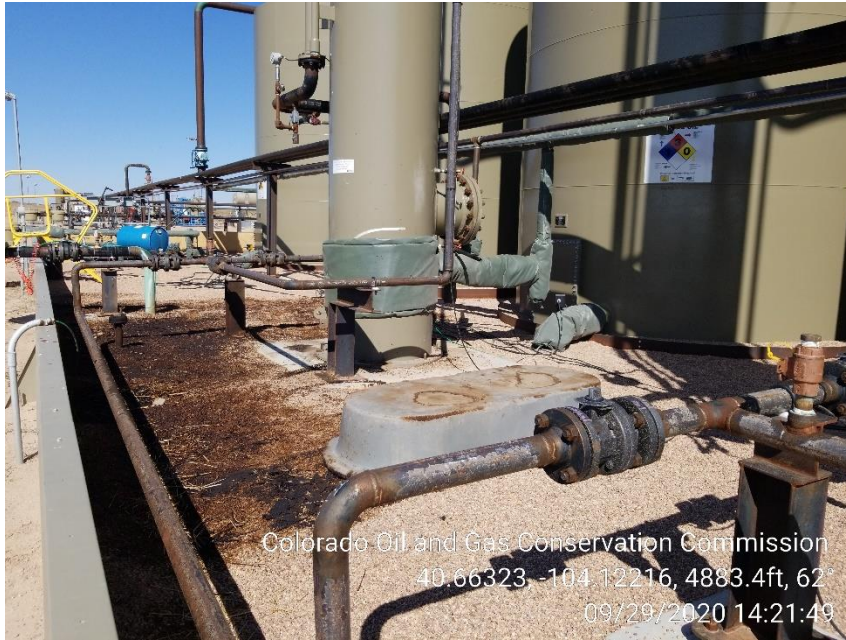
Photo 18 – Stained Soil at North VRT
