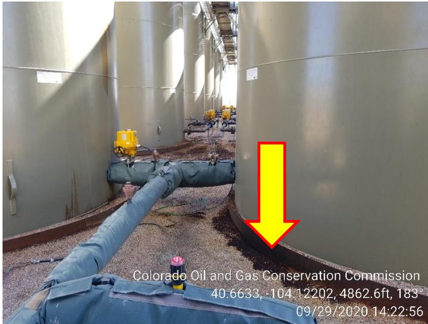
Photo 20 – Stained Soil at Tanks
