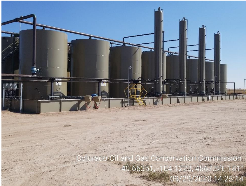
Photo 15 – Tank Battery and VRTs
