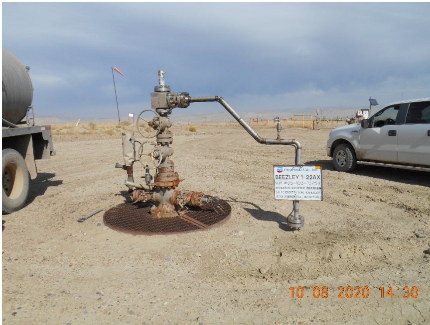
Injection wellhead
