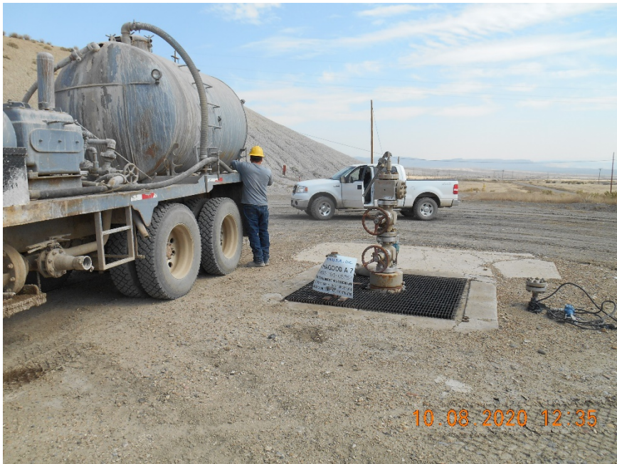
Injection wellhead
