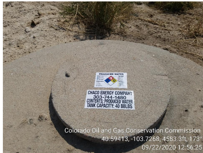
Photo 8 – Proper Labeling installed on Skim Tank
