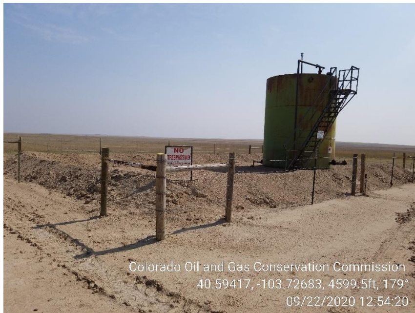
Photo 3 – Berms repaired and Barbed Wire Fence installed around Tank Battery
