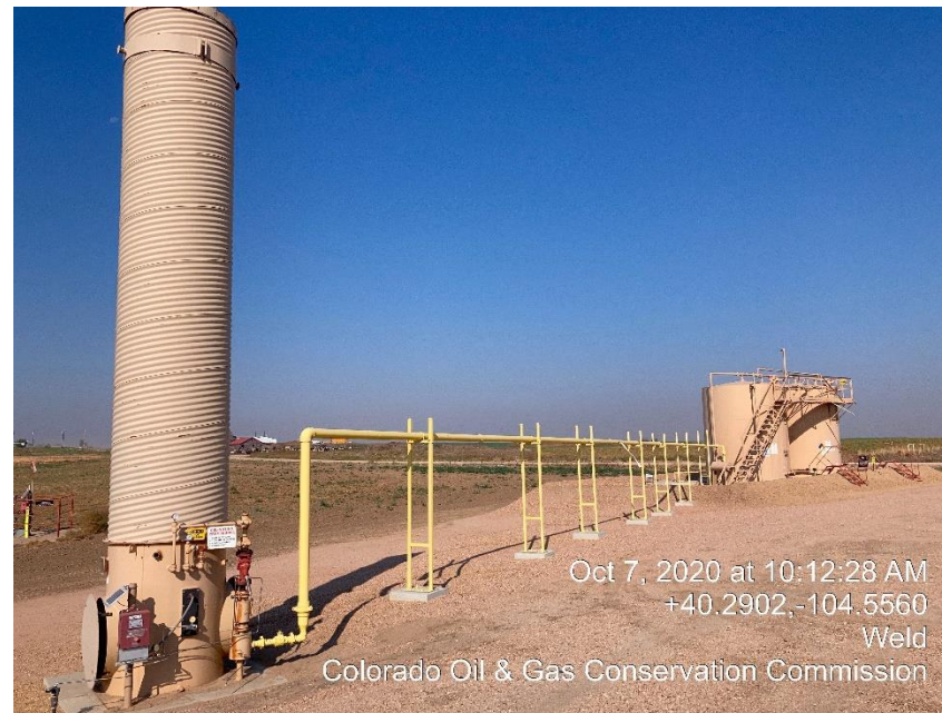
Photo #2 Tank Battery and ECD for Tanks
