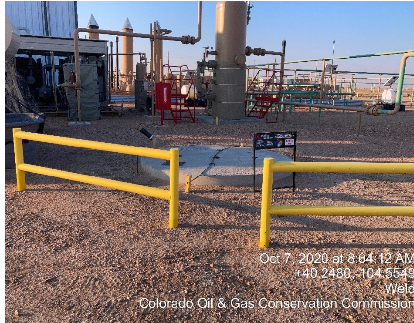
Photo #5 Pit needs secondary containment/ berms
