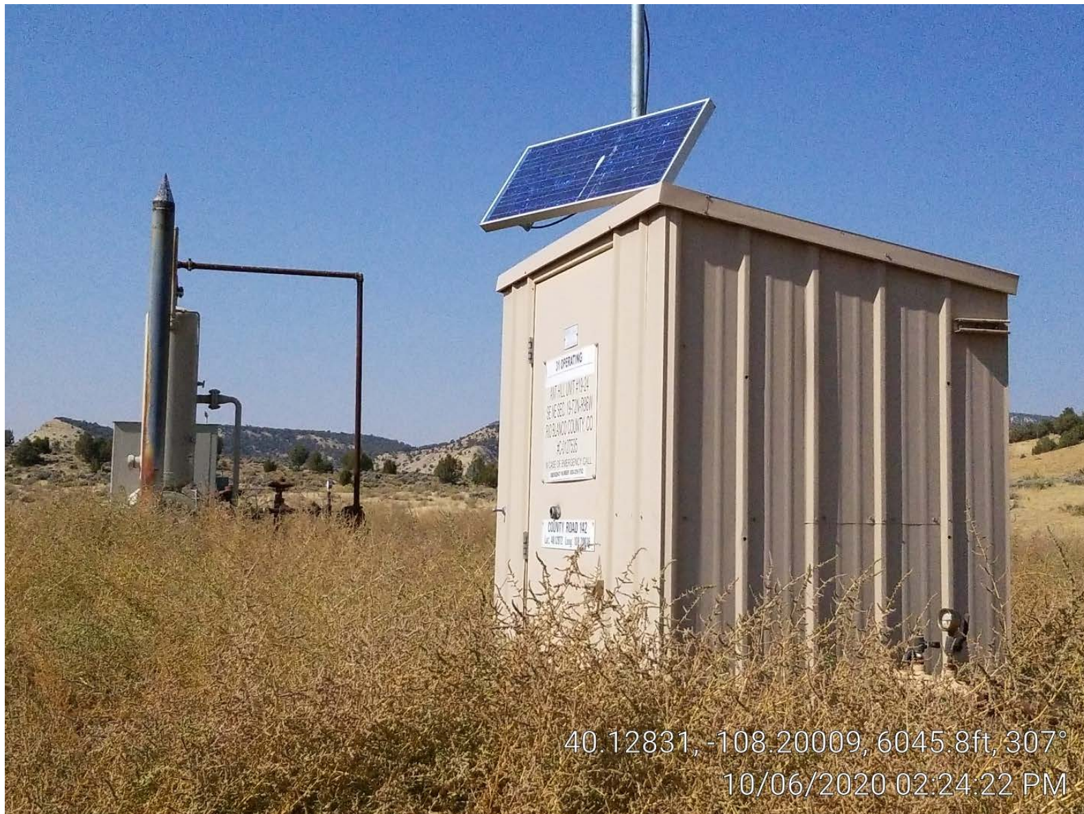
Photo 3. Meter building & separator.
